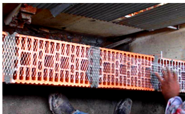
Step:2 Course Laying with GI Mesh application before bed mortar
