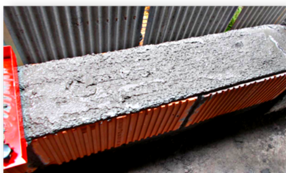
Laying Mortar
