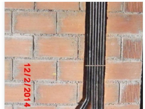
Step: 6 Placing pipes in the conduit
