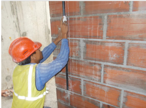
Step: 4 Nail the masonry joints
