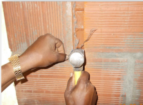
Step: 4 Nail the masonry joints
