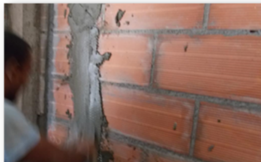
Step: 7 Pack the columns with mortar
