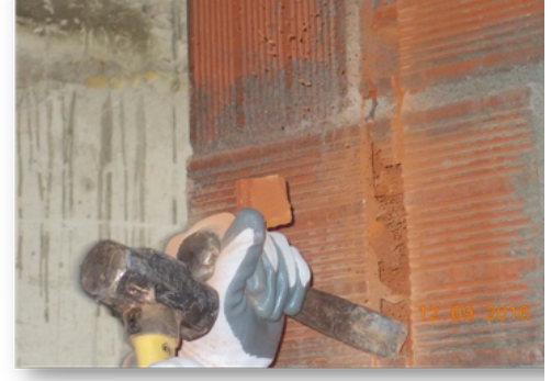
Step:3 Chip chased surface using hammer and chisel
