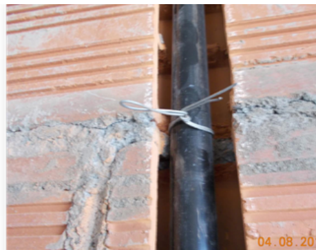
Step: 5 Place the pipes and tie them with binding wire
